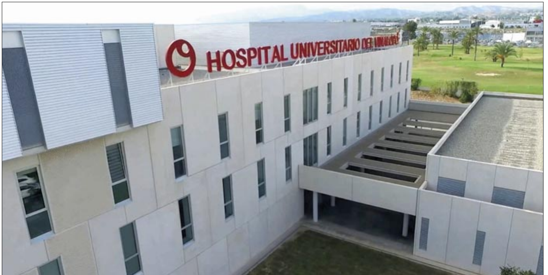
Vista general del hospital.
