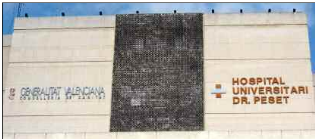
Vista general del Hospital.
