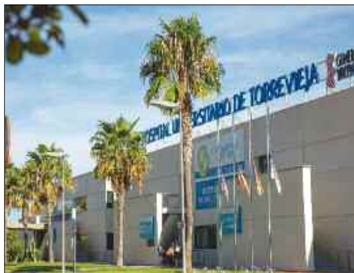
Vista general del hospital.
