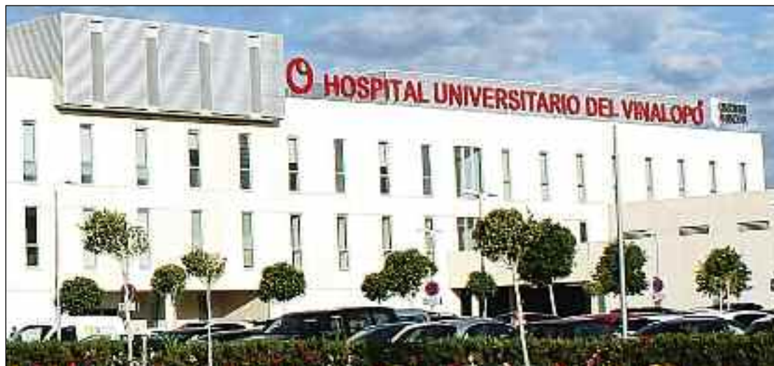
Vista general del hospital.
