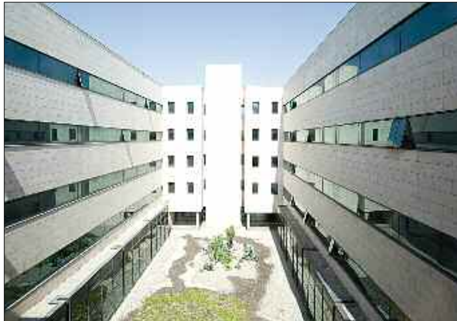
Vista general del hospital.
